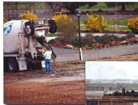
Figure 1. Chute washwater being dumped on the ground
