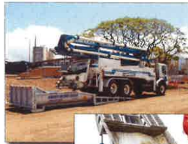
Figure 14. Pump truck using the ramp to wash out into a roll-off bin
