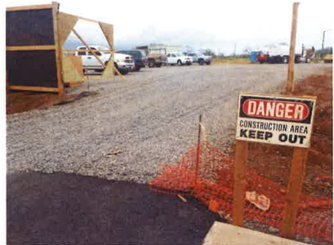
A construction entrance stabilized with gravel over filter cloth reduces the amount of sediment transported off site.
