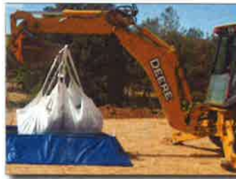
Figure 12. Extracting the concrete solids or gelled washwater
