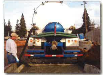
Figure 4. Vacuuming washwater out of a washout container for treatment and reuse
