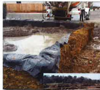
Figure 9. Hay bale and plastic washout pit
