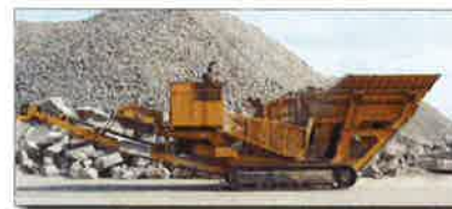
Figure 6. Crushed concrete stockpile and crusher
