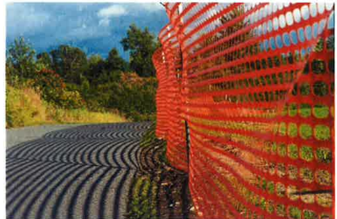
A construction safety fence preserves existing grass near a paved area.
