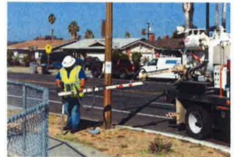
With the ERV-750 extended reach valve exerciser an operator can turn multiple nearby valves without moving the vehicle
