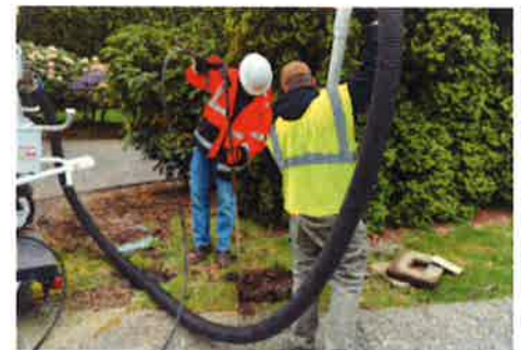
A two-person crew can excavate and vacuum debris from valve boxes for easy access
