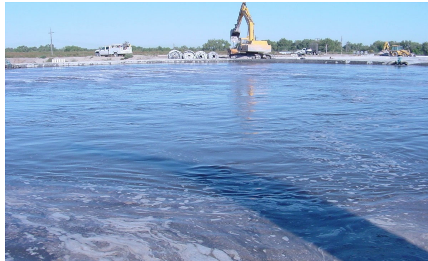
Wastewater Pond on U Street
