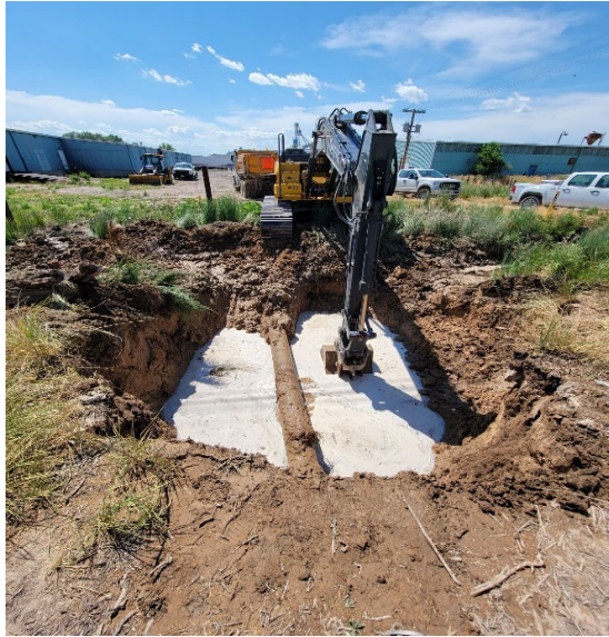
Water main repair on I Street
