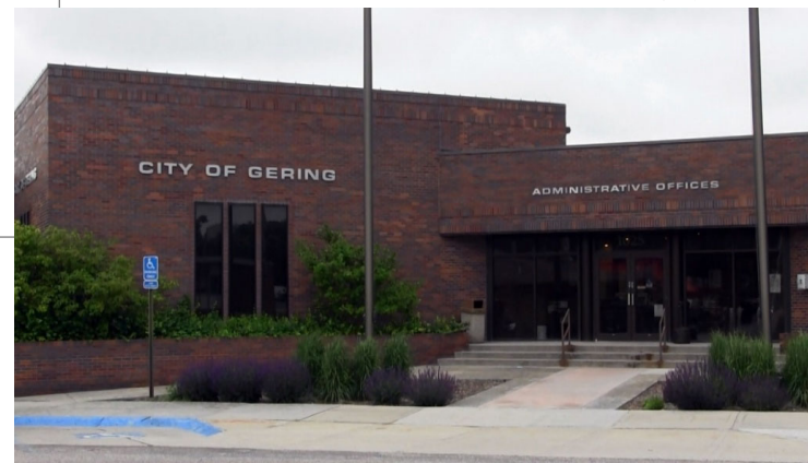
Gering City Hall - 1025 P Street
