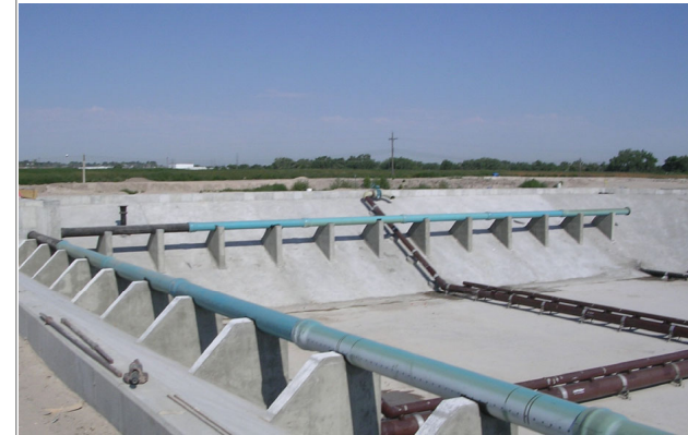
Waste Water Treatment Plant Aeration Basin
